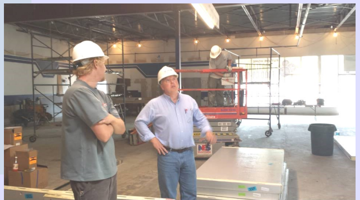
The Co-op hired the design-build team of Kaplan Thompson Architects and Warren Construction to lead the renovation effort.
